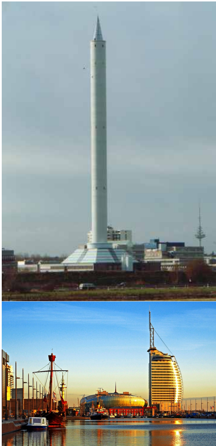
Figure 1.2: Upper panel: Drop tower in Bremen. Lower panel: Harbor in Bremerhaven, ca. 60 km north of Bremen.
